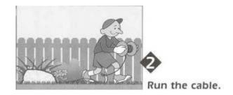
Before actually sinking the cable, run the cable from your unit to the power source or amplifier. Ensure your cable run avoids any obstacles such as sunken sprinkler pipes or piping and electrical cable to your house. Once the cable runs are where you like them, connect your speakers and power source to ensure correct operation <u>before</u> sinking the cable. Disconnect the cable wire at both ends and continue.
